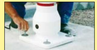
**STANDARD BOLT-DOWN FIXING**
