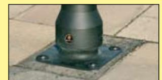
**THE BOLLARD FOOT CAN BE INSET INTO PAVED AREAS.** The top surface of the foot detail can be sunk level with the ground.
